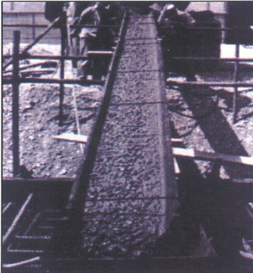
SCC placed using a Chute
