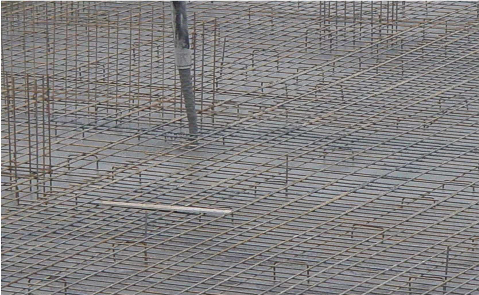
Casting a SCC Slab for a Commercial centre, Ferrara, Italy
