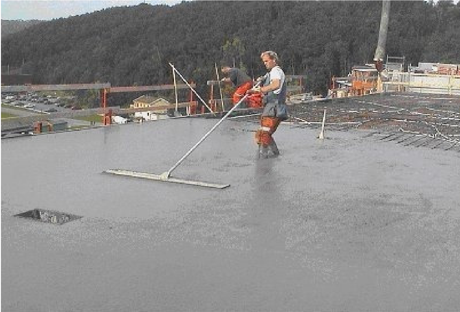
Levelling SCC with a Skip Float
