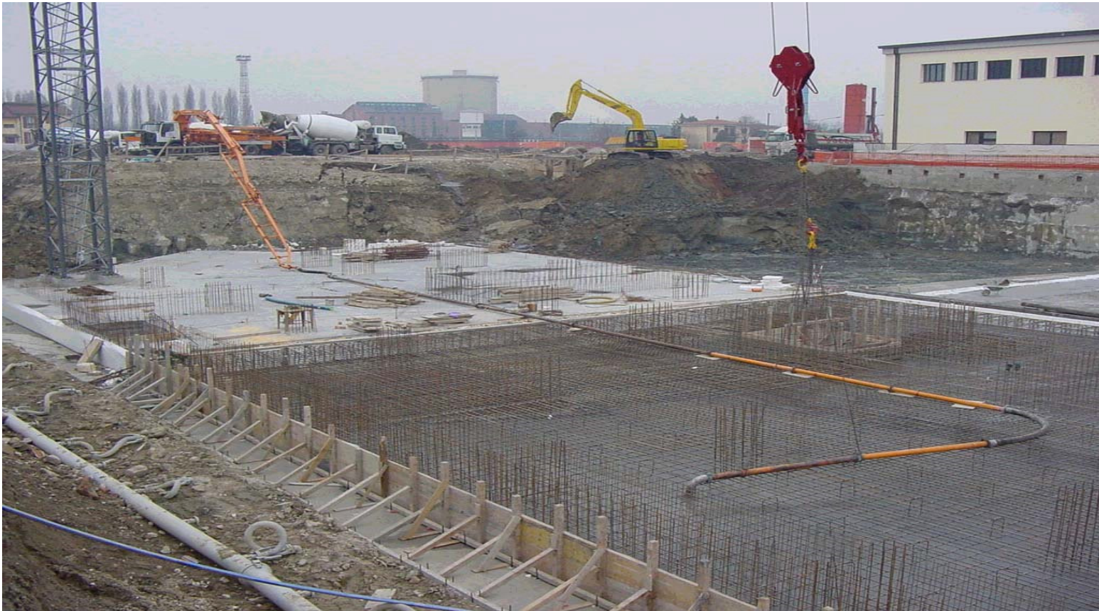
Casting a SCC Slab for a Commercial centre, Ferrara, Italy
