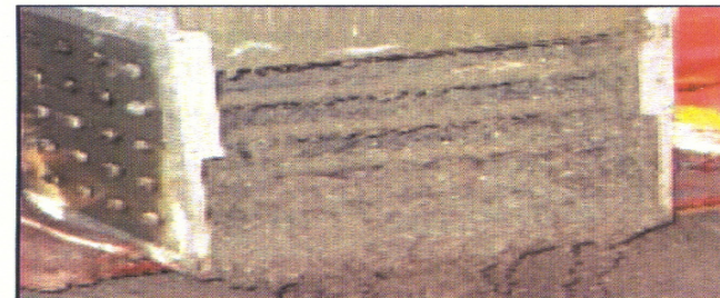
e) Concrete flows through the obstructions
